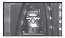
Unhook the gas meter and reinstall the port plug on the regulator.
